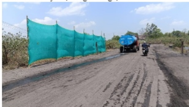
(Wind Barrier along road side at coal stock yard and Water Sprinkling from Mobile Tanker)
