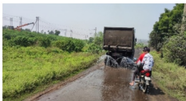
(Wind Barrier along road side at coal stock yard and Water Sprinkling from Mobile Tanker)
